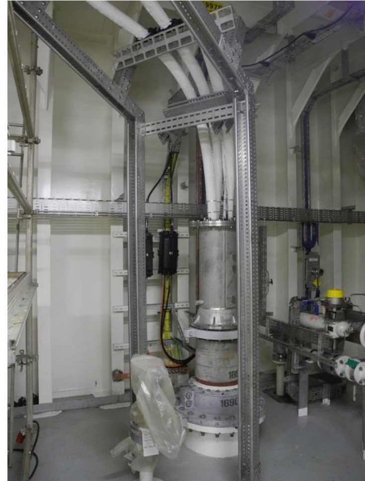
Power cable termination on FPSO
