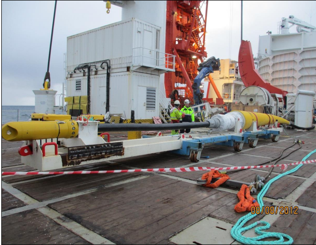
Power cable's FPSO end prior to installation
